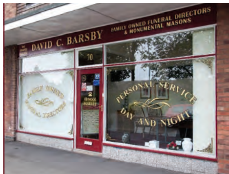
Newbold Verdon before renovation
